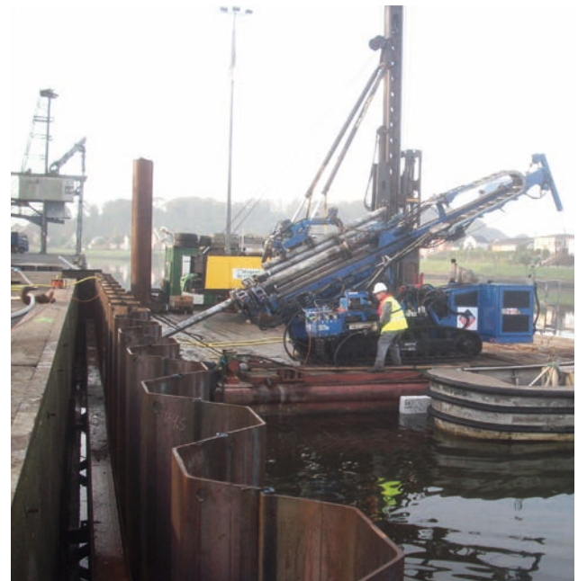
Image 1: Drill rig on a swimming platform
