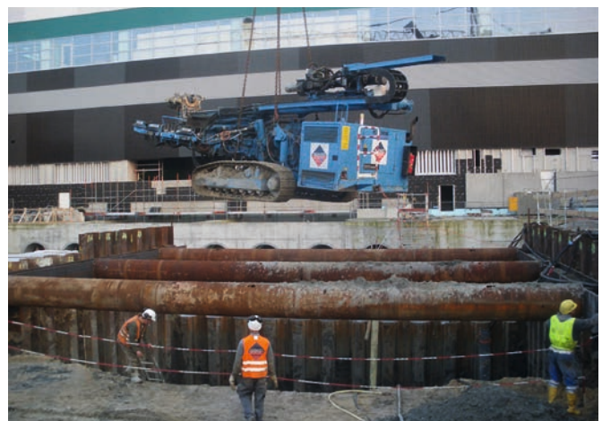
Image 1: Lifting our drill rig onto the work platform
