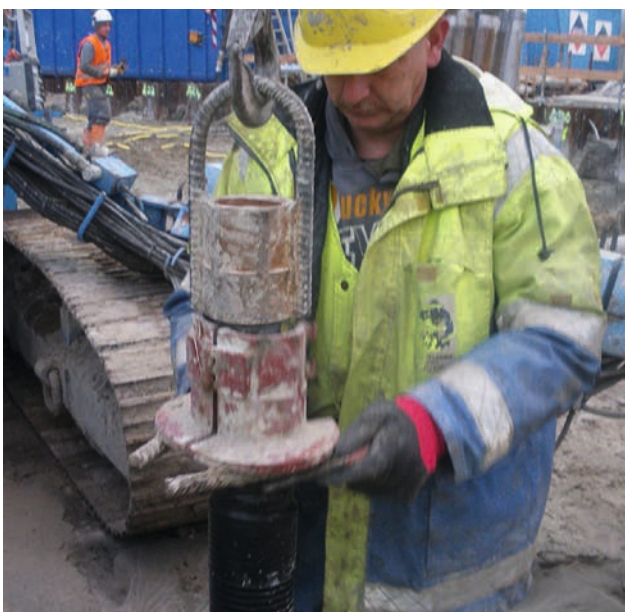
Image 2: Mounting a fold-out muffle to a GEWI-pile
